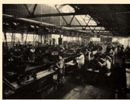
Tool room at the Birmingham site
